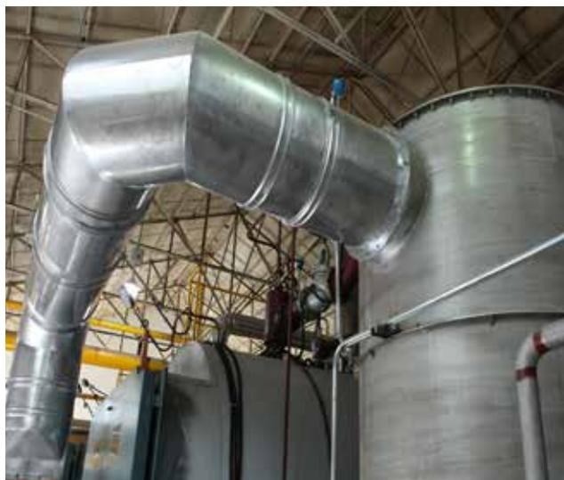
Figure 3. WVP combustion air spray tower
